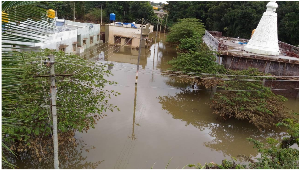
Fig.3: Image of the flooded area at Sai Layout, Kushalanagara.
